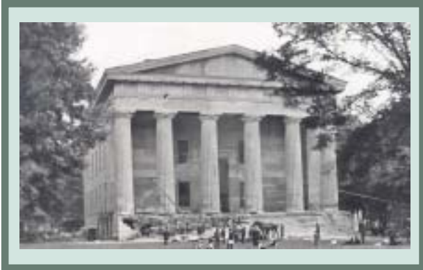
The New Haven State House being demolished
