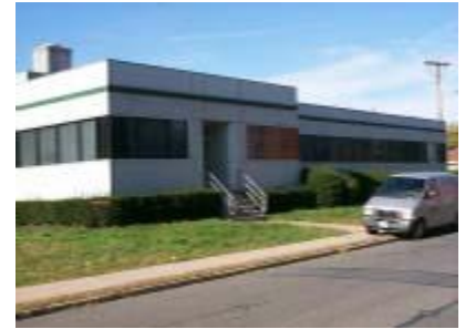
An exterior view
