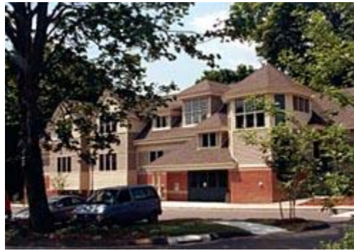
Douglas Library's new main entrance on the side Photograph furnished by Kenyon & Cutler Architects
